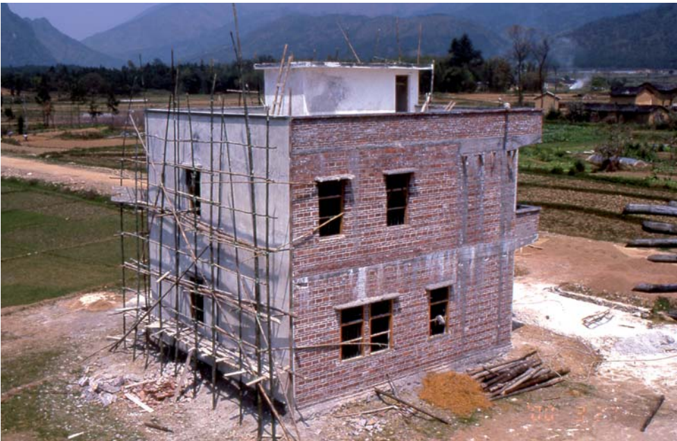
Fig. 12 A new village “mansion” (2005), Northern Guangdong. Photograph: Gonalo D. Santos.
